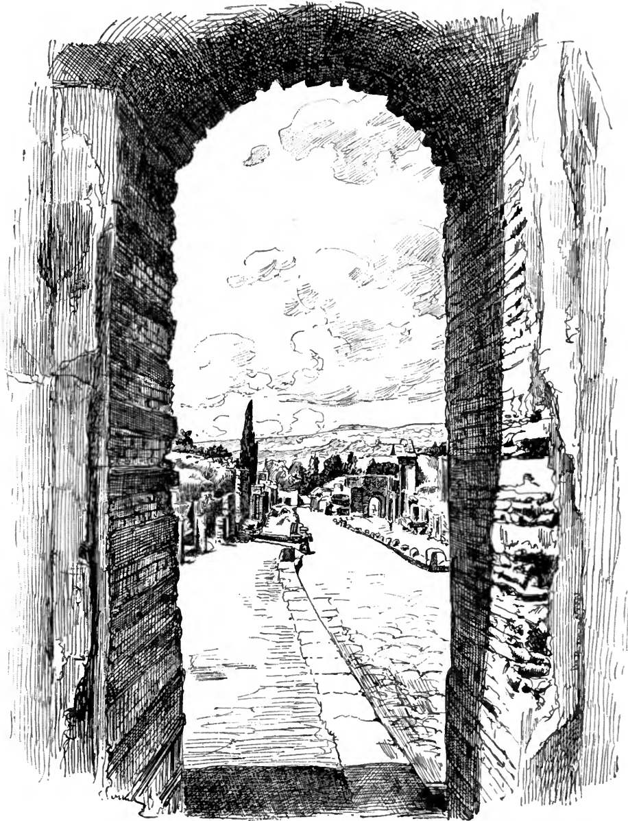
View from inside the Gate of Herculaneum
