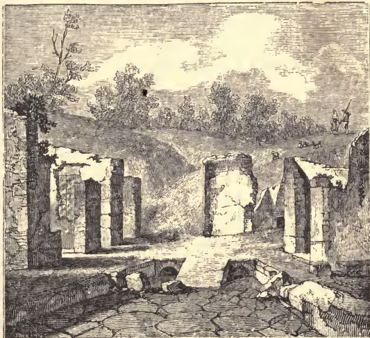
View of a Sewer in the city of Pompeii.
