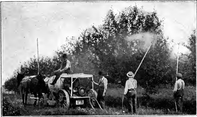
Fig. 60.—One of the many types of sprayers with power from a gasoline engine.
