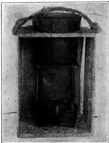
Fig. 11.—Handy method of heating grafting wax to paint wounds.
