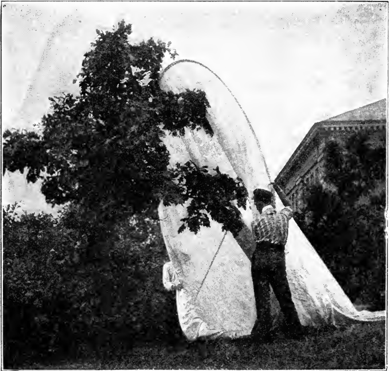
Fig. 37.—Hoop tent ready to put over a tree.
