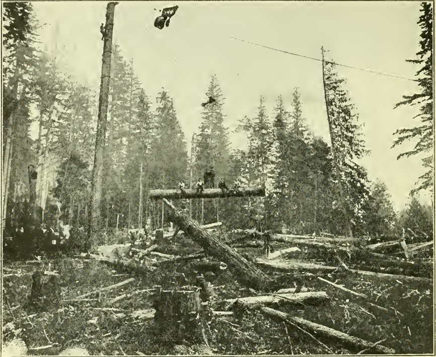
TRANSPORTING LOGS BY WIRE ROPEWAYS.
