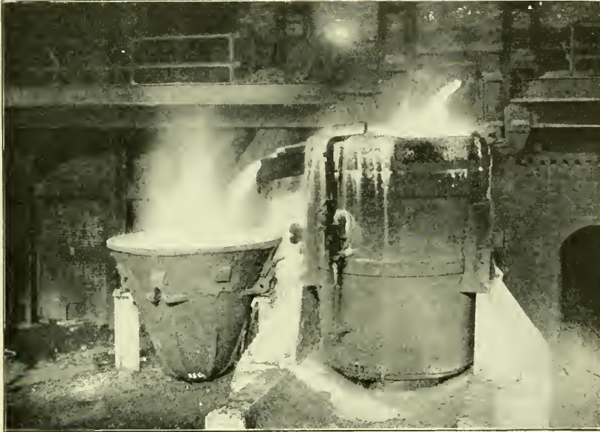
TAPPING AN OPEN-HEARTH FURNACE.
