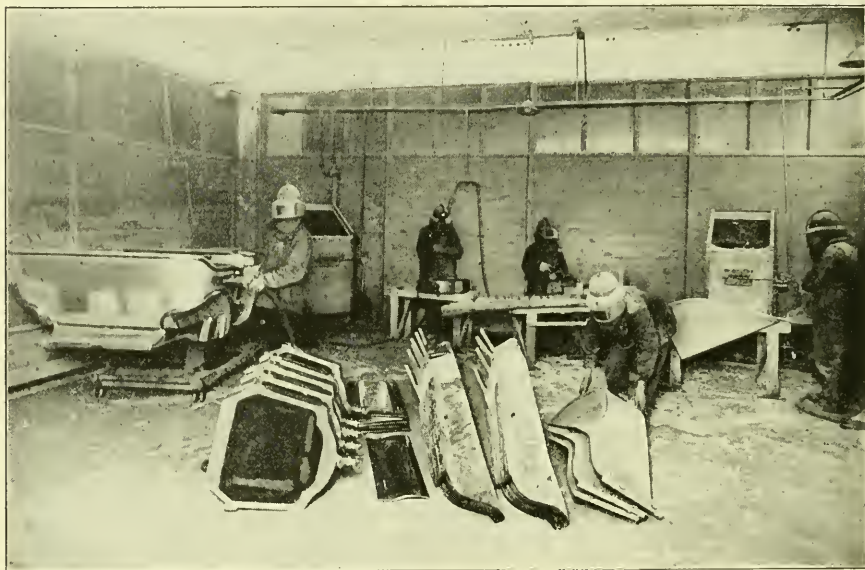
SAND-BLASTING SHEETS OF METAL MOTOR-CAR PARTS.
