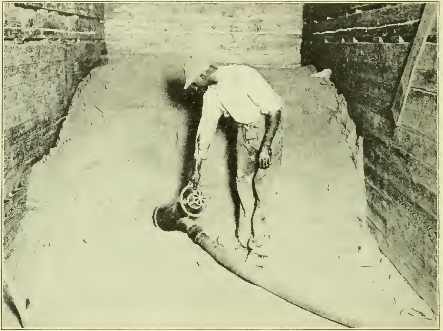
UNLOADING VERY FINE FERTILIZERS BY AIR FROM A BOX-CAR AT THE RATE OF TEN TO TWELVE TONS PER HOUR.
