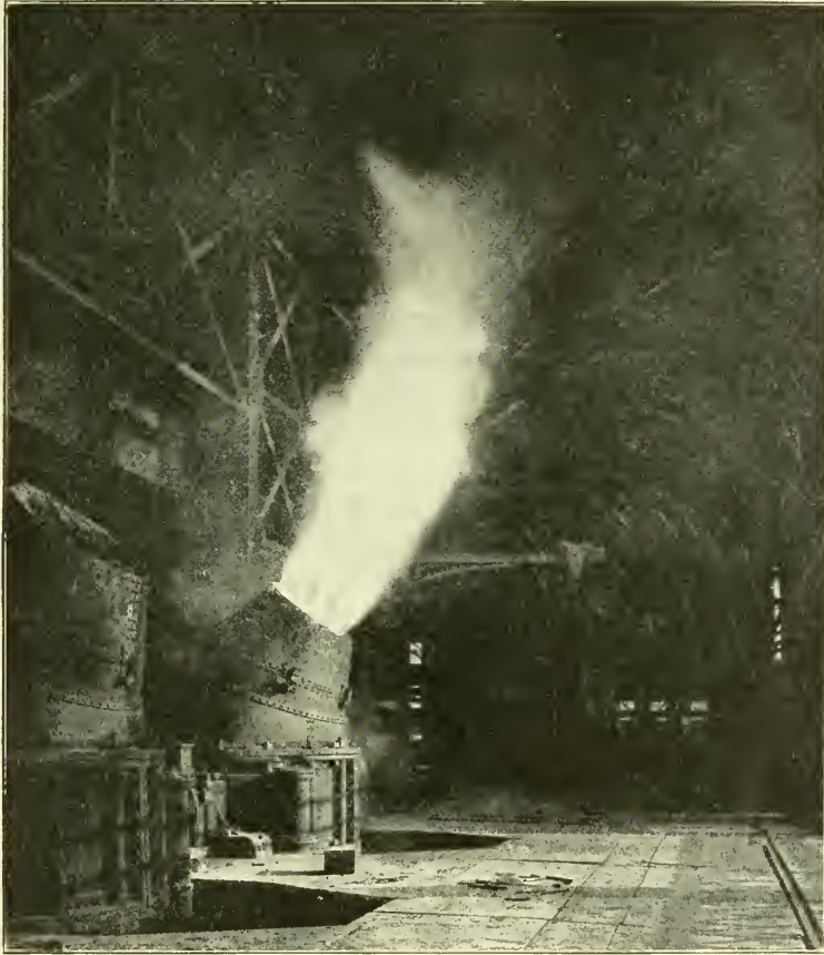
BESSEMER CONVERTER BLOWING OFF.
