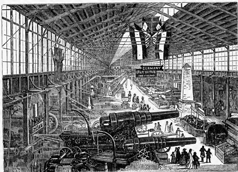
INTERIOR VIEW OF MACHINERY HALL.
