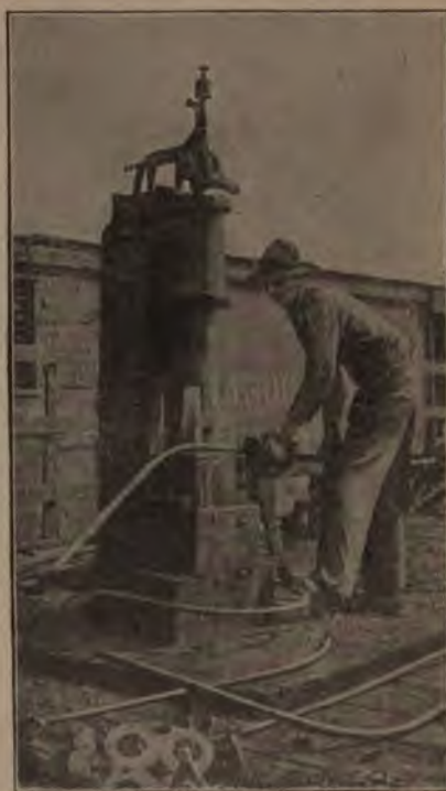
Air-Hammer for Straightening Scrap Iron.
