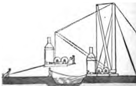
Moving the Hoisting Engine
