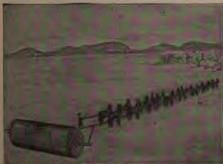
Mules Rolling the Boiler.
