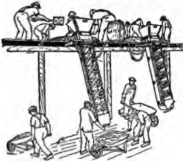
New Concrete Mixing Method
