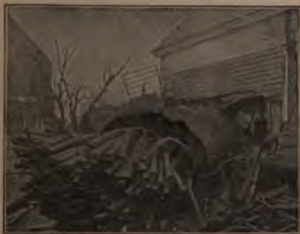
Brockton Lap-Joint Explosion--Boiler Was Hurlled 215 Ft. and Moved House 16 In.
