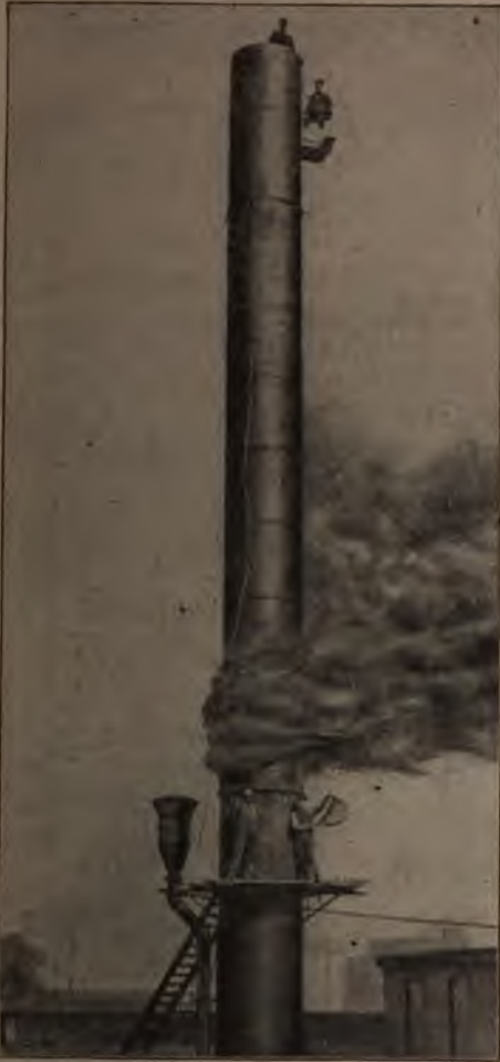
Lengthening a Stack While in Use
