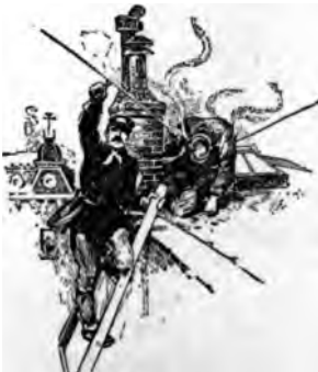
Rescuing from Contact with Live Wires.
