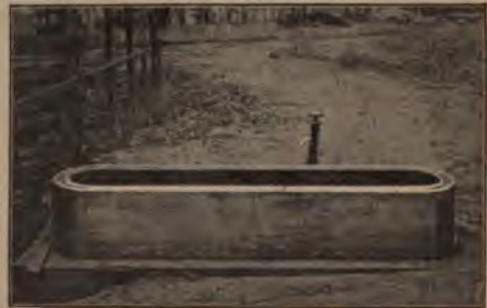
Side View of Cement Trough.
