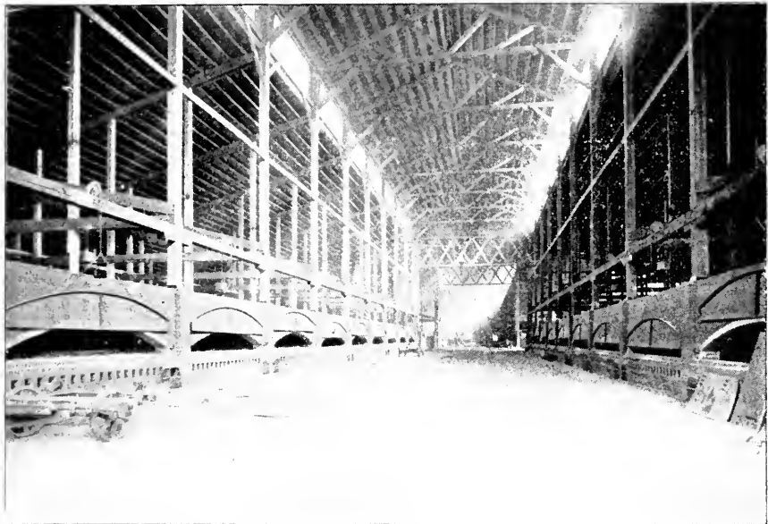
INTERIOR VIEW OF THE CASTING HALL AT FORD CITY, PA.
