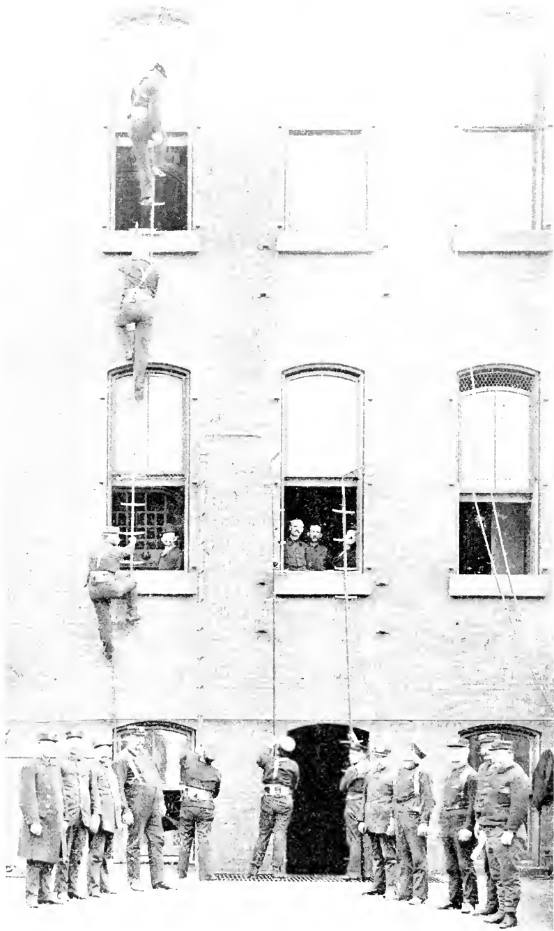
FIG. 22.—SCALING A BUILDING WITH FIREFIGHTER LADDERS.
