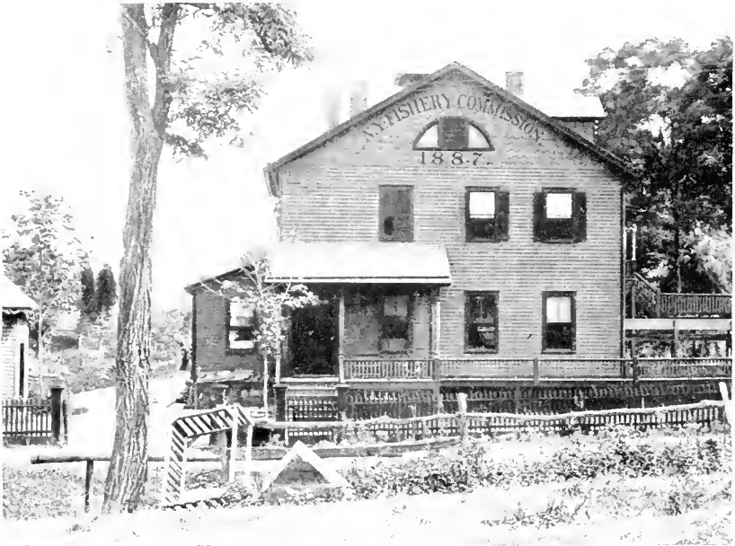
FRONT OF HATCHERY, SHOWING INLET TRUNK FROM RESERVOIR.
