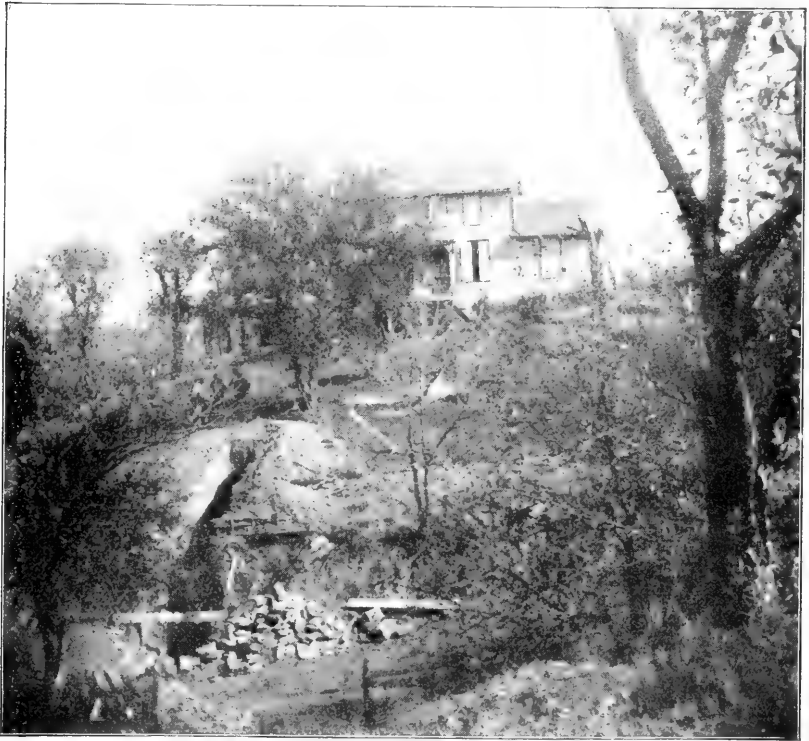
VIEW FROM THE WEST SHOWING INTERSECTING TRENCH DUG TO JOIN THE ORIGINAL TUNNEL, with the Concannon residence in background. The skeleton was found nearly below the place indicated by the larger light spot at the right of the trees. From a photograph by Professor Chamberlin.
