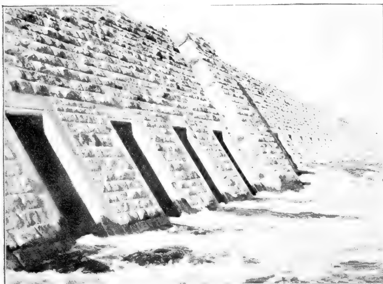
FIG. 3. NORTH SIDE OF DAM, LOOKING WEST.
