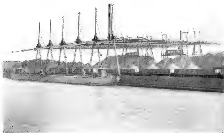
BRIDGE TRAMWAYS FOR HANDLING ORE AND COAL. MENOMINEE DOCK AT ASHTABULA.
