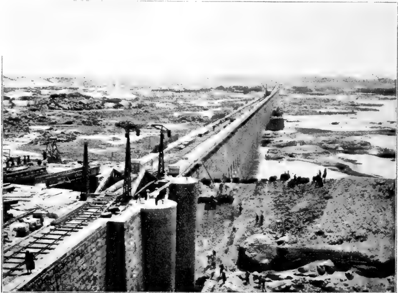
FIG. 4. SOUTH SIDE OF DAM, FROM WEST BANK.
