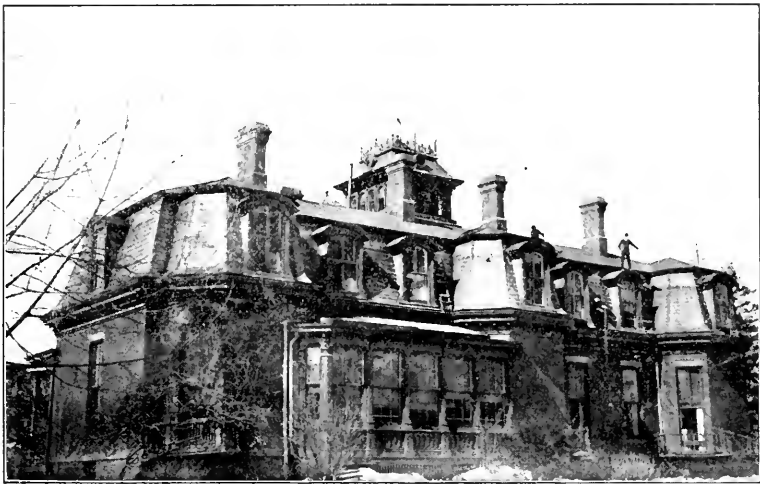
HIGH SCHOOL BOYS ATTACHING WIRES TO POLE placed on the cupola of the Children's Museum Building for Wireless Telegraphy.
