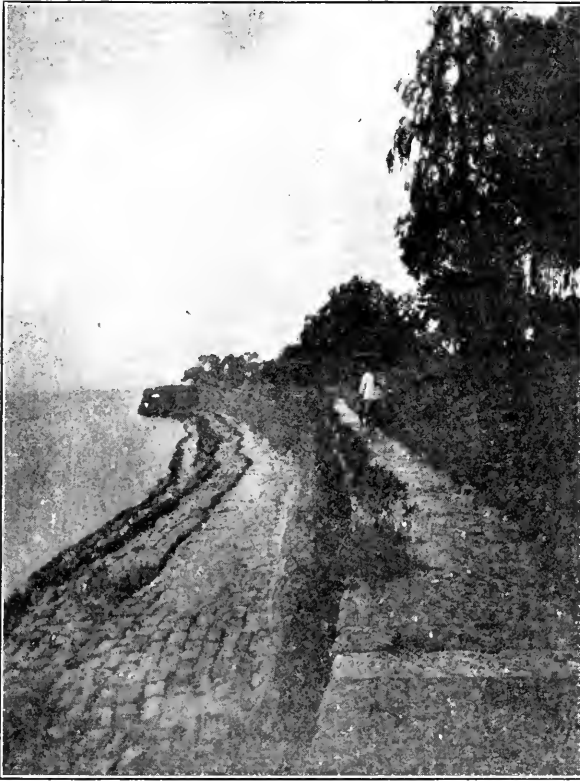
VIEW FROM THE TOP OF THE SEA WALL, SHOWING THE SUCCESSIVE LEDGES OF THE SEA-FOOTING AND A BUFFER IN THE DISTANCE.
