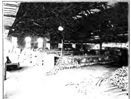
ELECTRIC FURNACES OF THE RESISTANCE TYPE IN WHICH ARTIFICIAL GRAPHITE IS MADE.
