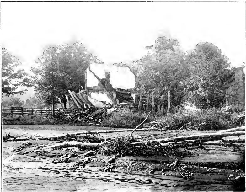
THE RUINS OF A BRICK HOUSE DEMOLISHED BY THE FRESHET OF MAY 21, 1901. BAKERSVILLE, MITCHELL CO., N. C.
