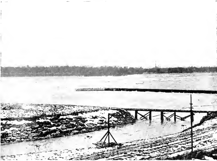
FIG. 3. PROFILE OF RIM OF FIRST CASCADE, with forebay of Ontario Power Company in foreground.
