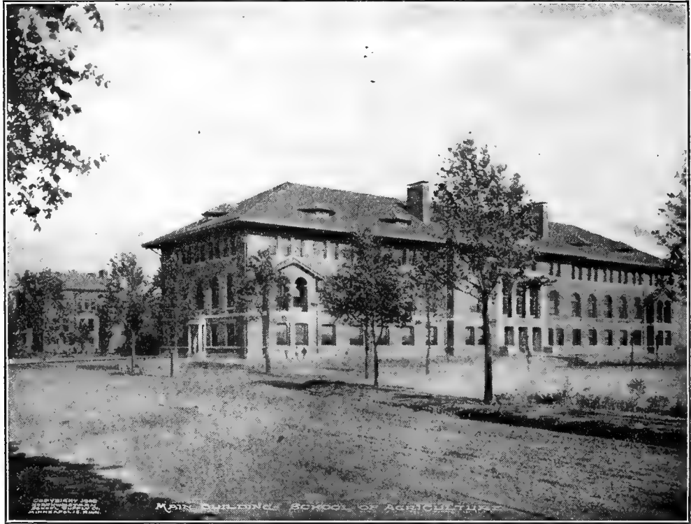
MAIN BUILDING OF THE SCHOOL OF AGRICULTURE.
