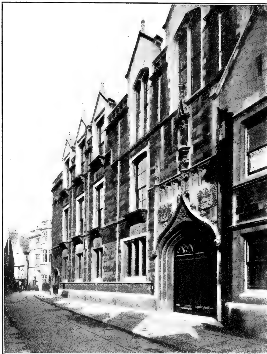
ENTRANCE OF CAVENDISH LABORATORY, SHOWING EXTENSION IN THE DISTANCE.
