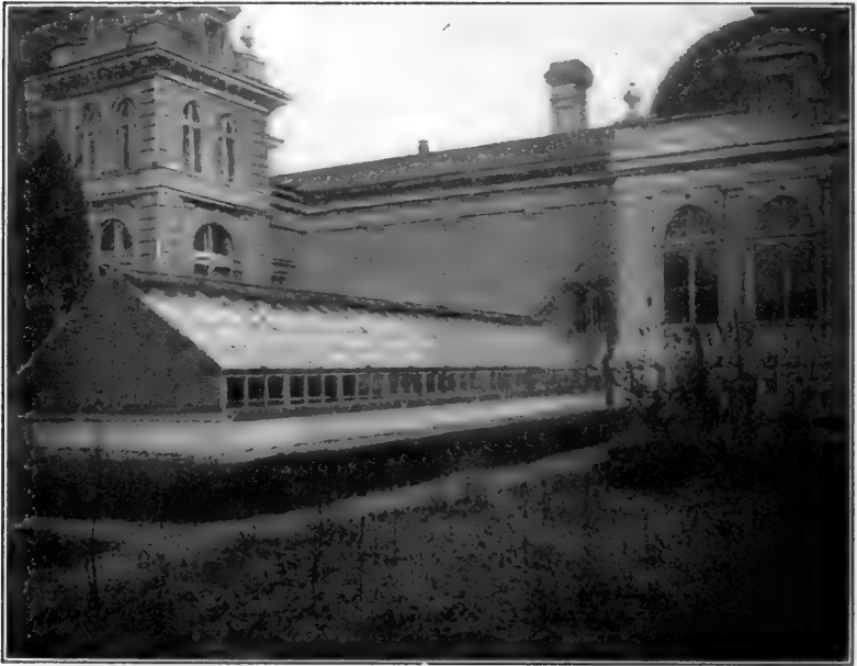
FIG. 5. VIEW OF THE GLASS HOUSE FOR LOW TEMPERATURES.
