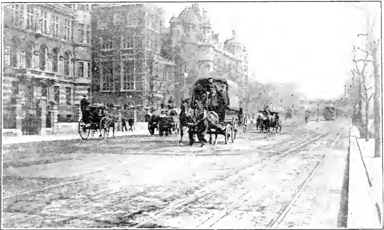
VICTORIA EMBANKMENT, LONDON. Paved with Trinidad Lake Asphalt in 1906.
