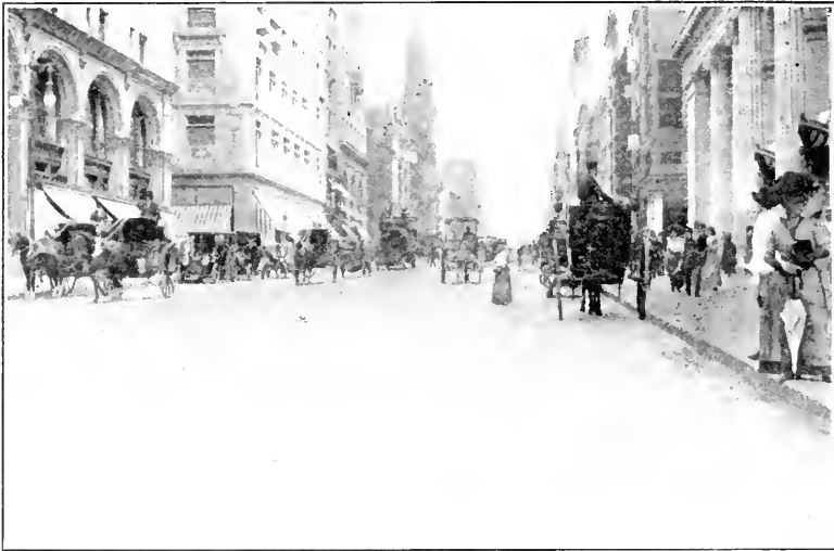
FIFTH AVENUE AT 34TH ST., NEW YORK CITY. Paved with Trinidad Asphalt 1897, photographed 1911.
