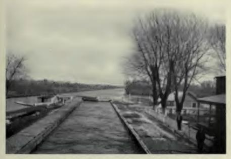
An Example of the Obsolete Type of Canal Lock, Limiting Traffic.
