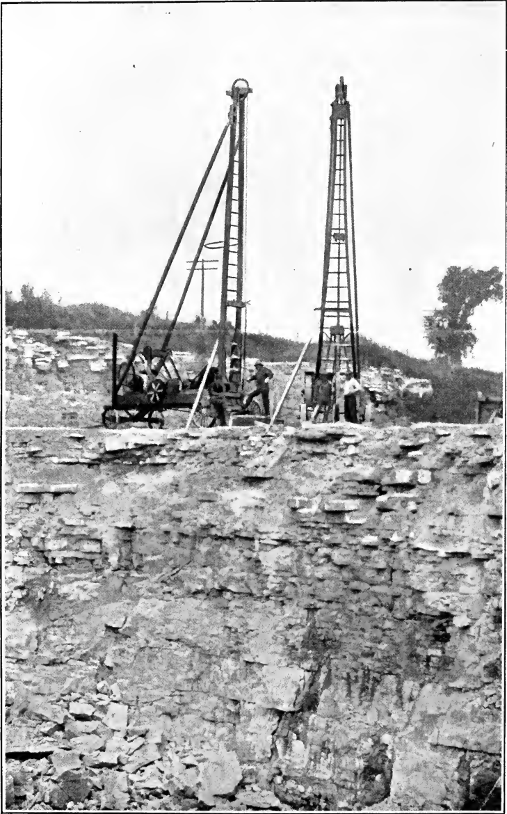
BIG BLAST HOLE DRILLS IN OPERATION.
