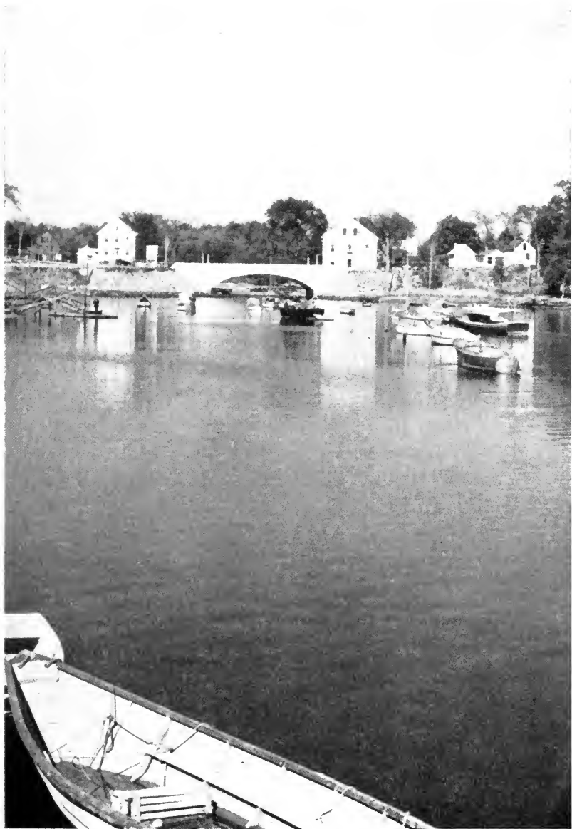
Bridge at Yarmouth
