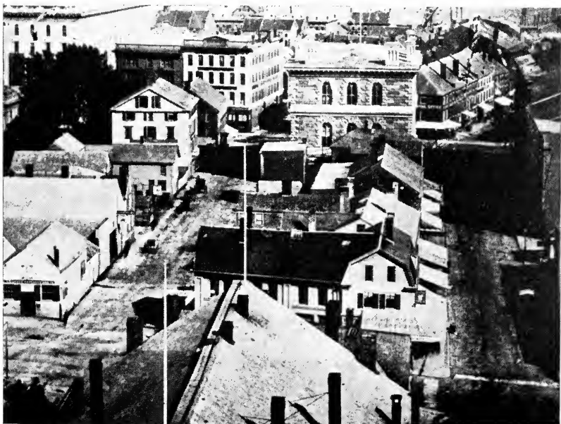
View down Exchange and Lime (Market) Streets (1862)
