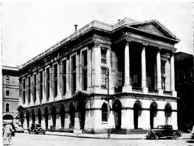
Old Post Office Building
