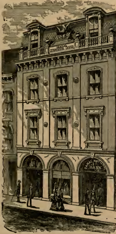
CANAL BANK BLOCK.
