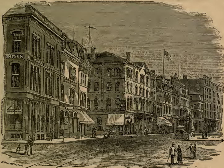
LOOKING UP MIDDLE-STREET FROM THE POST-OFFICE.
