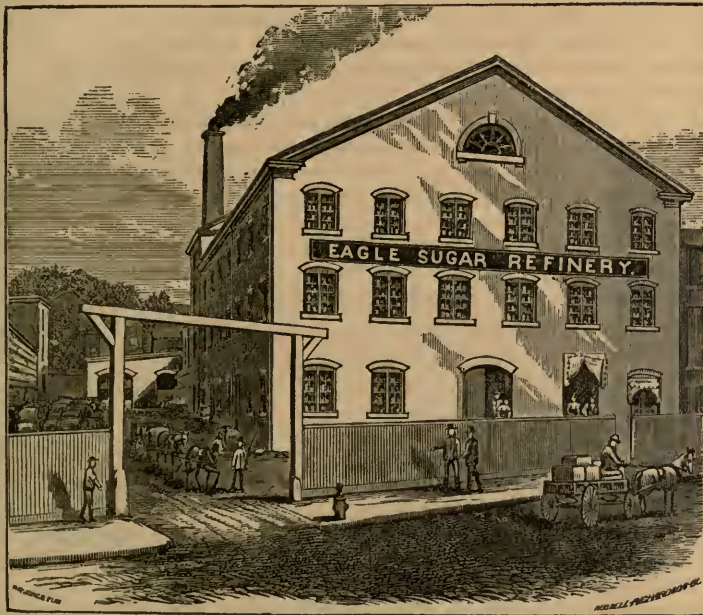
EAGLE SUGAR REFINERY.
