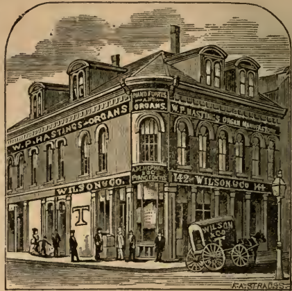
VIEW COR. EXCHANGE AND FEDERAL STS.
