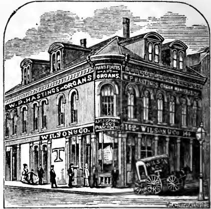
VIEW COR. EXCHANGE AND FEDERAL STS.
