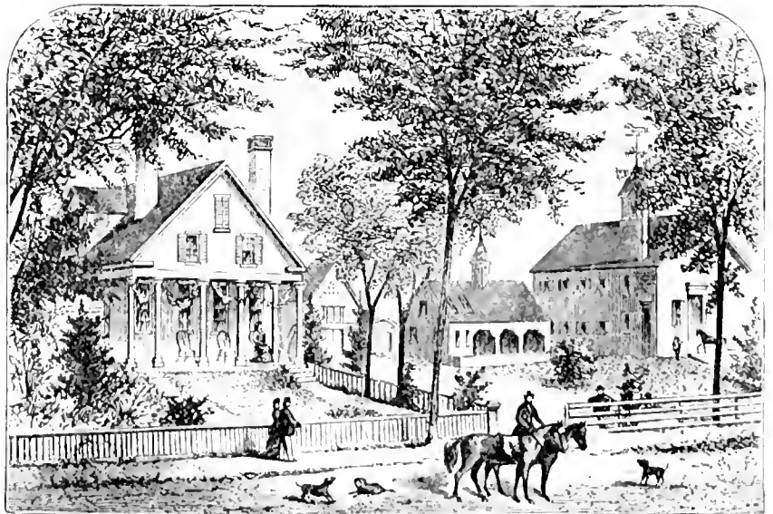
Civic Cottage. Former Residence of Dr. Tewksbury
