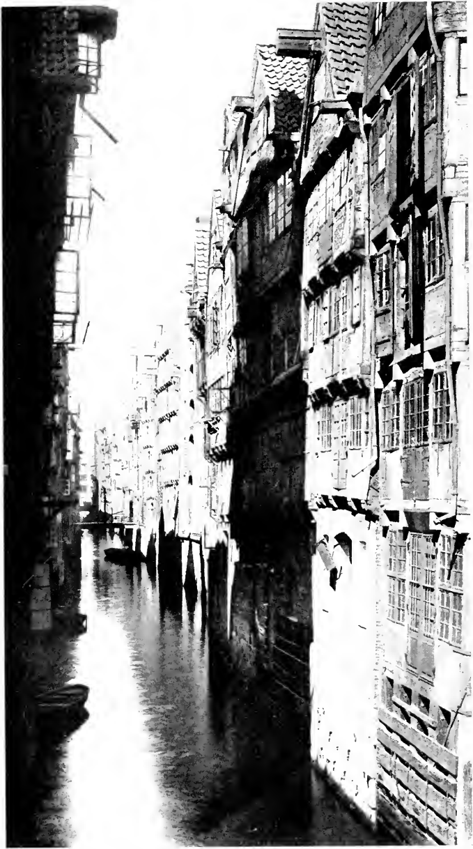
A row of old warehouses on the Steckelhorn, one of Hamburg's ancient canals.
