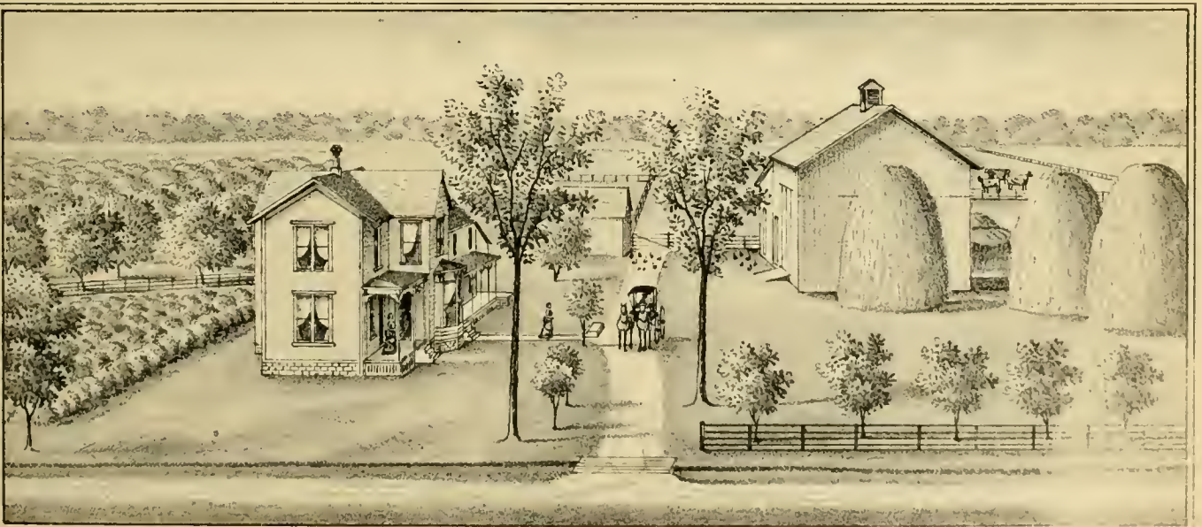
RESIDENCE OF JAMES HUBBARD, SEC. 3., BINGHAM TP., CLINTON CO. MICH.
