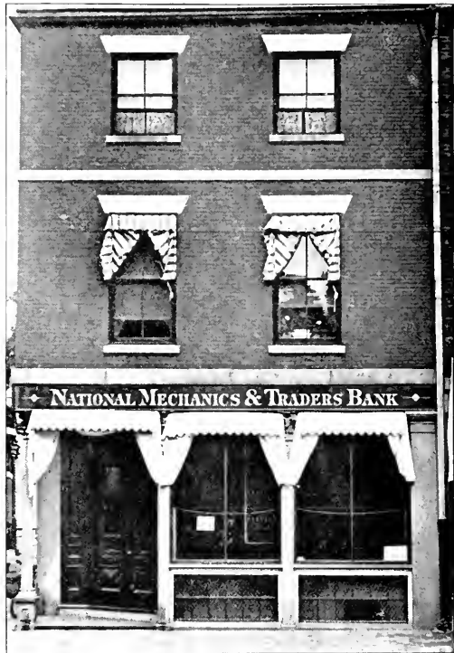
NATIONAL MECHANICS & TRADERS BANK BUILDING.
