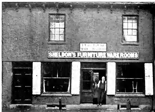
OLD POST OFFICE 1829 - 1840, NOW SHELDON'S FURNITURE ROOMS.
