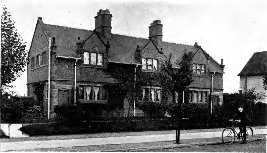
GREENDALE ROAD COTTAGES.
