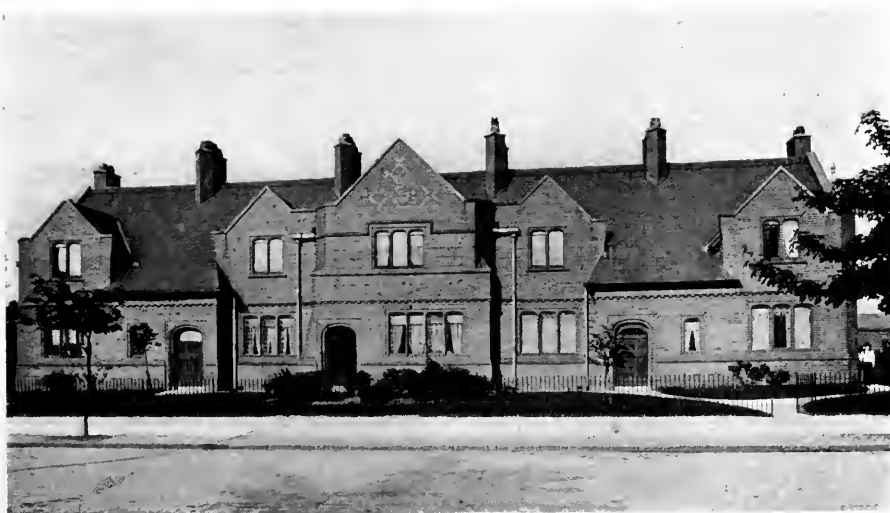
GREENDALE ROAD COTTAGES.
