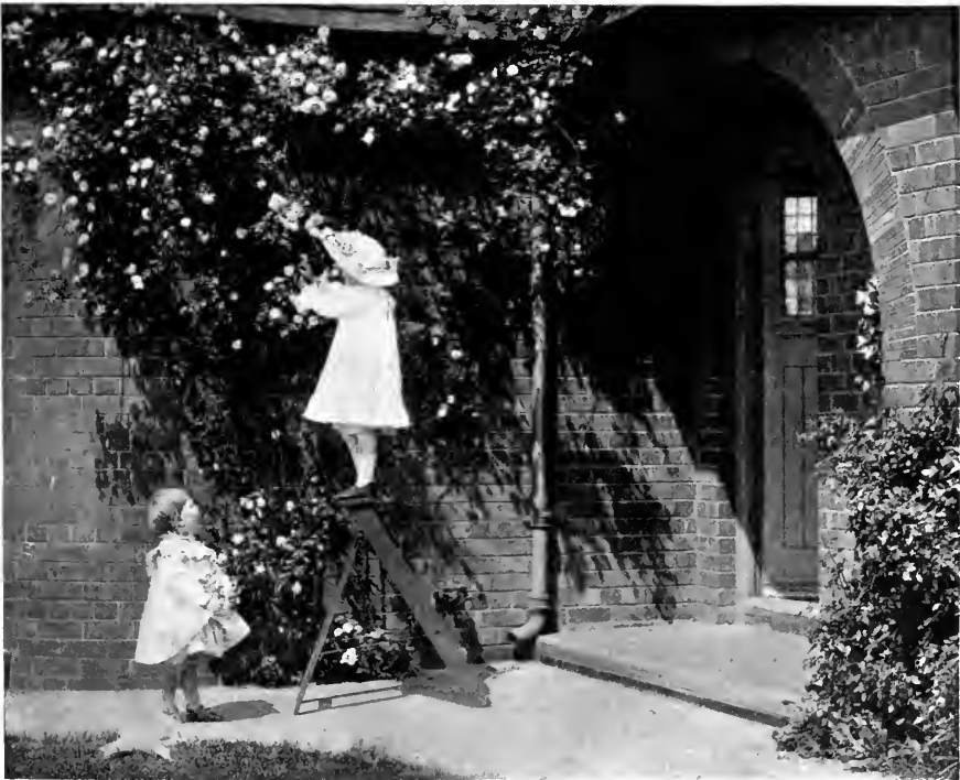
COTTAGE PORCH, CONNOLLY ROAD.
