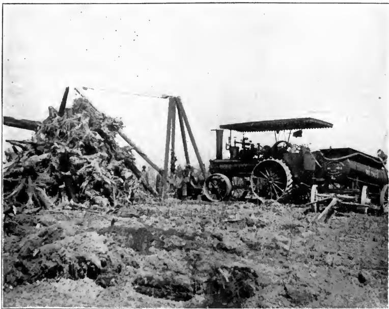
PULLING AND PILING STUMPS BY STEAM POWER AT STARKS ONEIDA COUNTY.
