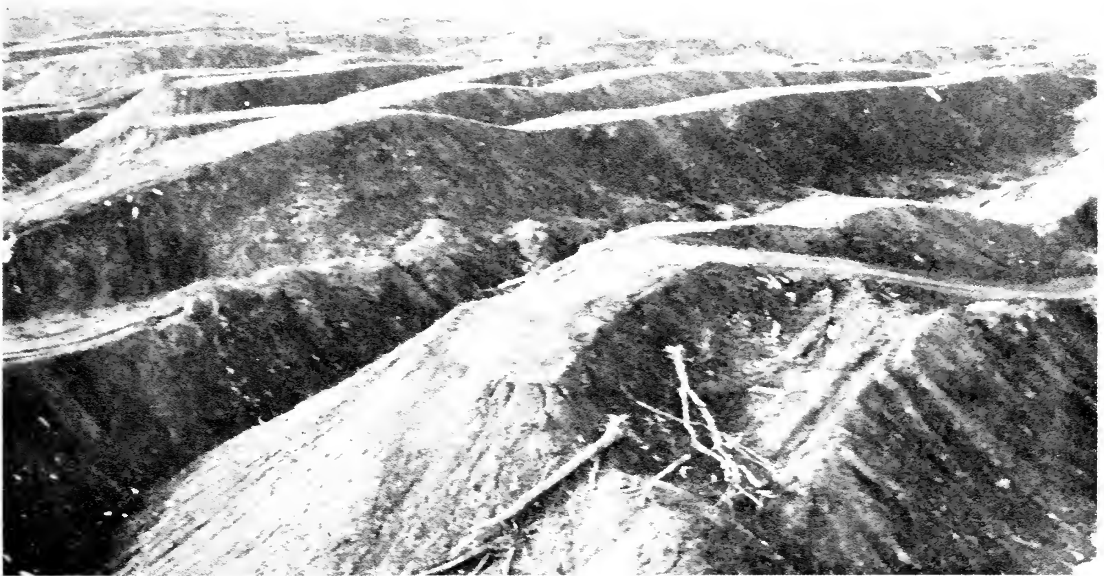
Spoil bank ridges struck-off to a width of 12-16' by means of a bulldozer. Fairview Collieries Corporation, Fulton County. (Fig. 6)
