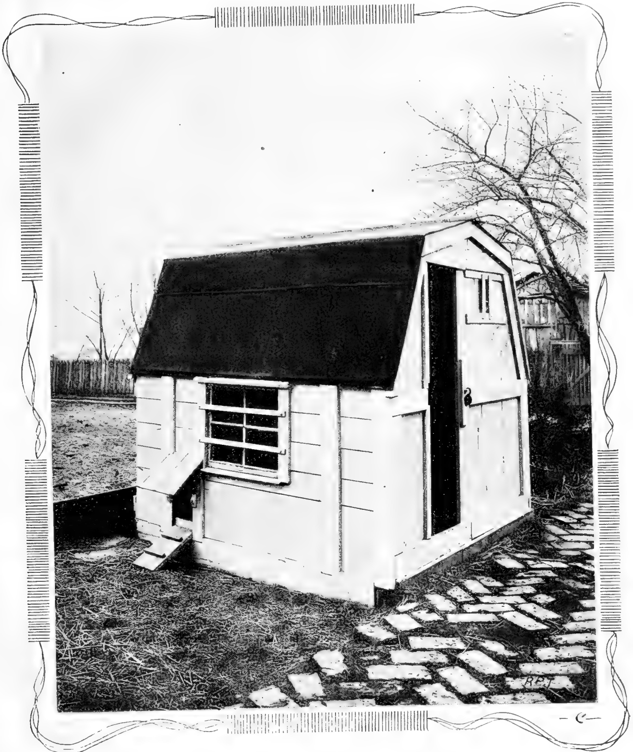
PIANO BOX POULTRY HOUSE
