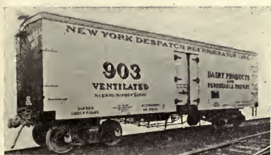
FIG. 21.—Refrigerator car used for shipping dressed poultry and eggs. An important factor in widening the market for the Western poultry keeper. (U. S. Department of Agriculture.)
