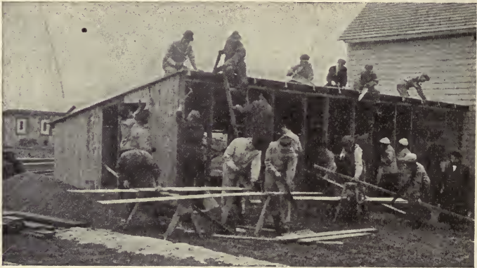
FIG. 3.—Students constructing a poultry house.
