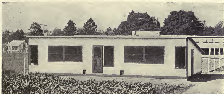
FIG. 85.—Double-unit house completed. Note the combination door and window, and the arrangement of openings for light and ventilation.
