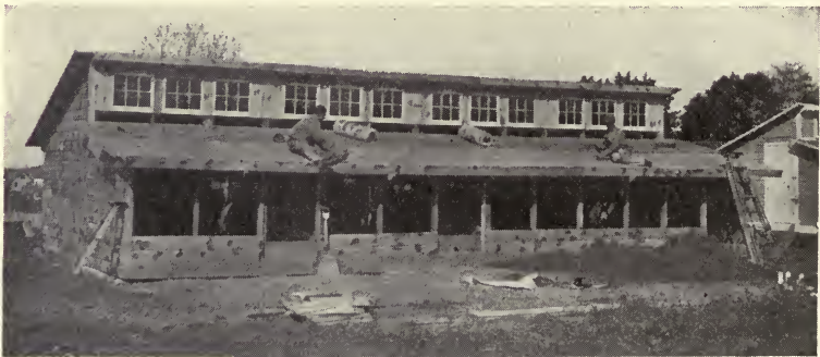
FIG. 91b.—Half-monitor type of laying house*: Under construction
