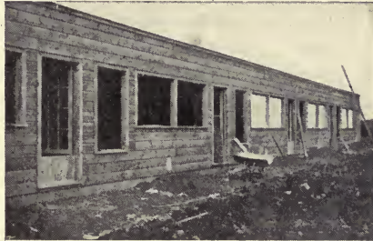
FIG. 65.— Modern type of poultry house with both muslin and glass in front, providing an abundance of light and ventilation without drafts.
