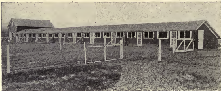
FIG. 89.—Laying house with two-thirds span roof. A neat house. The cost is greater and the front lower than with the shed roof.
