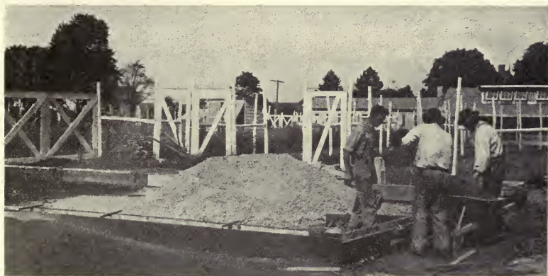
Fig. 82.—Placing fresh concrete in completed forms for foundation wall.
