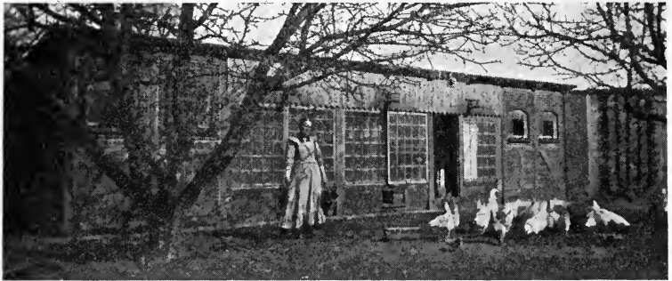
FIG. 28.—A typical Danish poultry house. A roosting room is at each end with a glass-front scratching shed between. Brick is commonly used.
