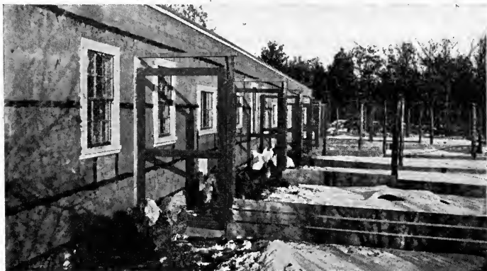
FIG. 64.—Antiquated type of poultry house, with no muslin in windows. Glass prevents ventilation and holds the moisture.
