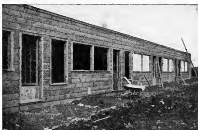
FIG. 65.— Modern type of poultry house with both muslin and glass in front, providing an abundance of light and ventilation without drafts.
