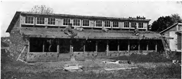
FIG. 91b.—Half-monitor type of laying house*: Under construction
