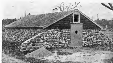
FIG. 19.—Incubatorcellar in the South Shore district, Mass., showing economical construction with field stones laid in mortar. (Photo by E. O. Damon, owner.)
