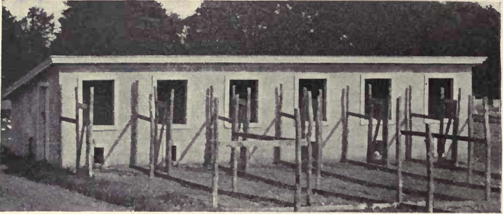
FIG. 113.—A poultry house built of hollow tile and stucco. This material costs just about one-half more than the same house would have cost built of wood.
