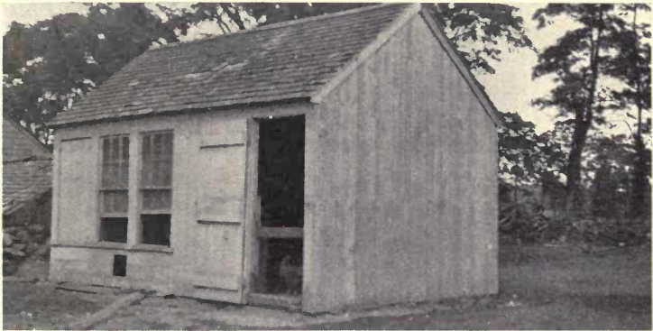
FIG. 120.—A type of gable or even span poultry house which is especially common in southern New England.
