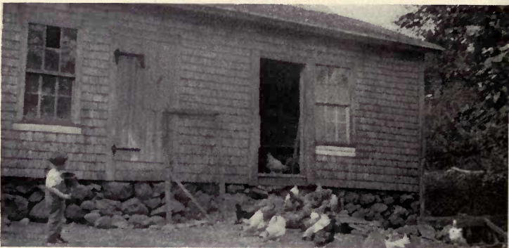
FIG. 93.—The boiler room of an old grist mill was remodelled into a poultry house for twenty-five birds so that the little man might have a place for a special flock all his own.
