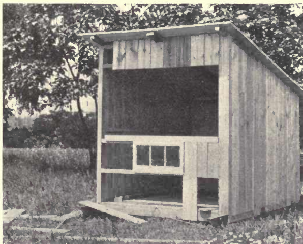
FIG. 102.—Boarding up the walls. Note openings left for muslin curtain, window and exit for the birds.
