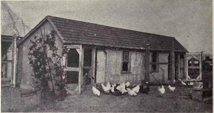
FIG. 119.—A double-pen, scratching shed, laying house with a broken or two-thirds span roof.
