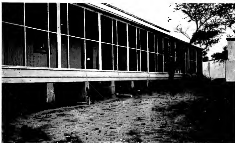
1. AN EXCELLENT TYPE OF MOSQUITO-PROOF HOUSE AS BUILT BY THE TRANSVAAL GOVERNMENT.
