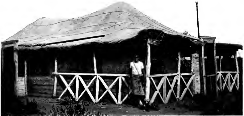
2. AN EXAMPLE OF ROUGH BUT EFFICIENT MOSQUITO PROOFING IN THE VELDT. A hut at Sabi Bridge, Game Reserve, Transvaal, formerly occupied by the Warden, Major Hamilton.
