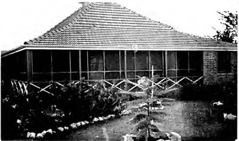
4. A GOOD EXAMPLE OF MOSQUITO-PROOF HOUSE. The Customs quarters, Komatipoort.
