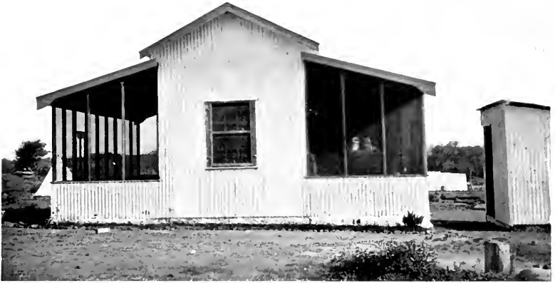
TWO-ROOMED WOOD AND IRON HOUSE WITH MOSQUITO-PROOF VERANDA. As built by the C.S.A.R. for temporary quarters at the Sabi Bridge, Selati Railway. Cost about £180.
