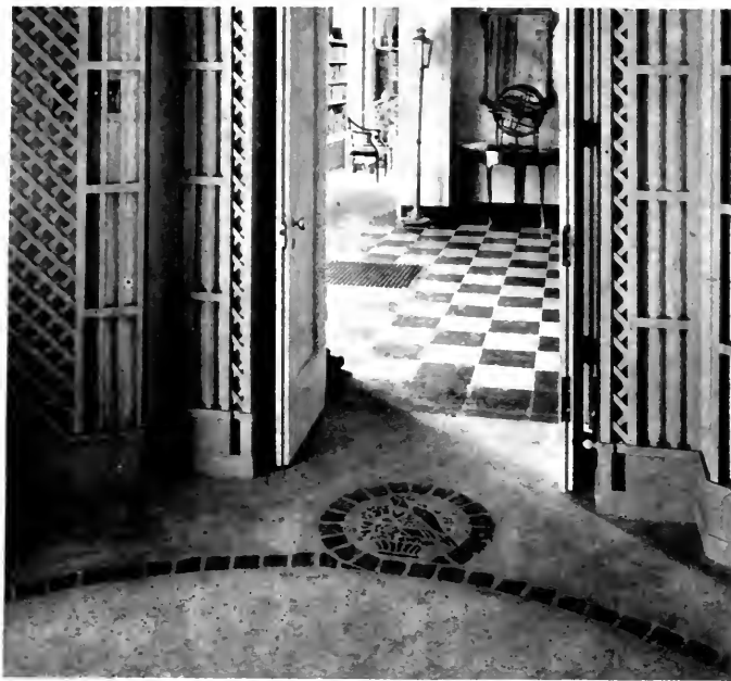
A. CEMENT FLOOR WITH INSERTED DESIGN IN COLOURED TILE By Courtesy of George Howe, Architect
