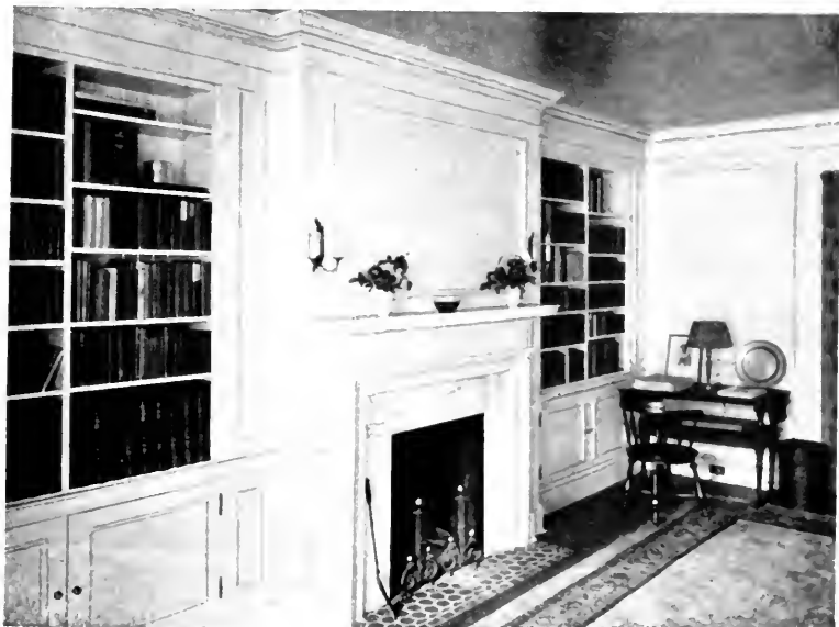
B. WALLS COVERED WITH FILLED CANVAS, AND MOULDING APPLIED TO FORM PANELS
