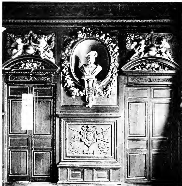
WOODWORK AND PLASTERWORK, GALLERY, FONTAINEBLEAU. STYLE FRANCIS I
