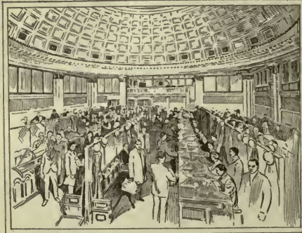
INTERIOR VIEW OF A CLEARING HOUSE.
