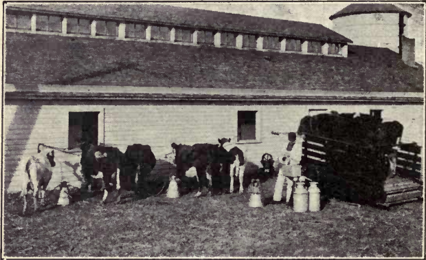
FIG. 54—USE OF A MILKING MACHINE OUT OF DOORS Power is supplied by animals in treadmill on right (Kansas Experiment Station)
