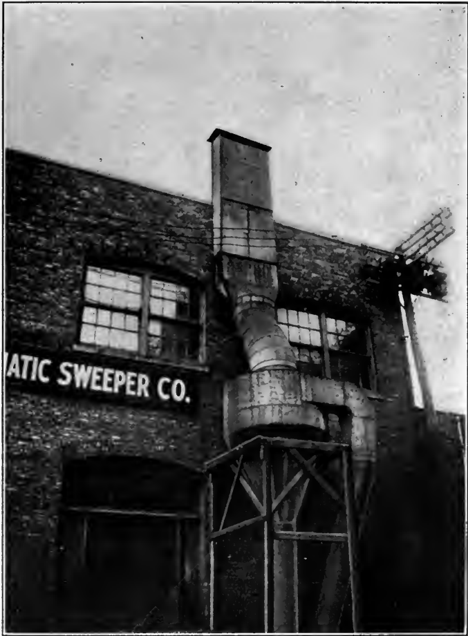
FIG. 187.—A problem in sheet metal work, involving nearly every problem in Descriptive Geometry, including the intersection and development of plane, single-curved, and warped surfaces. The picture itself is a problem in shades, shadows, and perspective.
