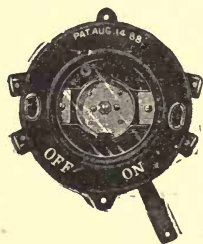
FIG. 42.—ARC CUT-OUT SWITCH.
