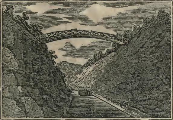
Deep Cut of the Chesapeake and Delaware Canal.
