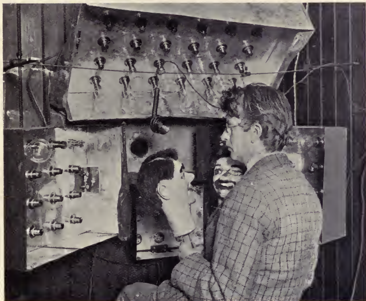
FIG. 91.—Bank of Lamps.
