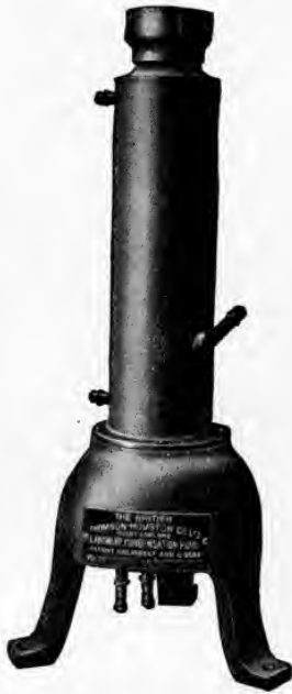
FIG. 38.—The Langmuir Mercury Vapour Pump.
