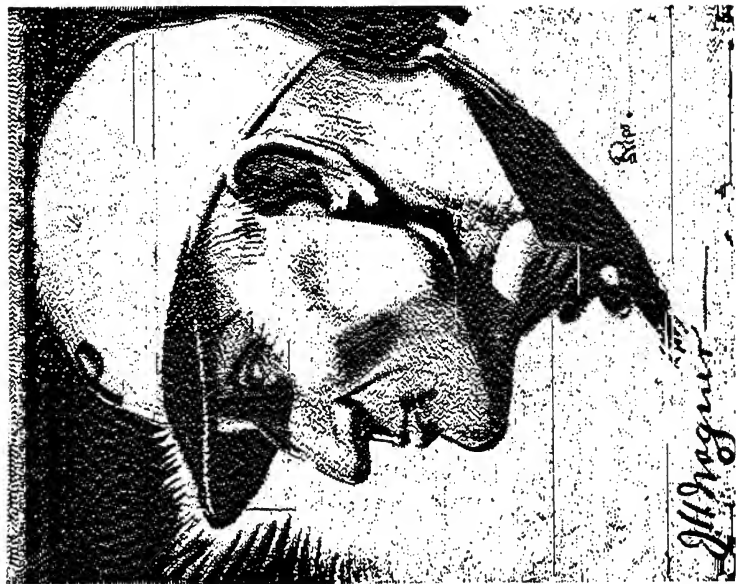
FIG. 2.—Specimen of a Drawing of a Baseball Player transmitted between New York and London by Radio.
