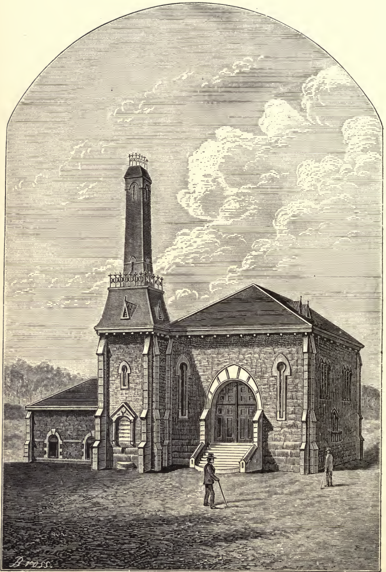
PUMPING STATION, NEW BEDFORD.
