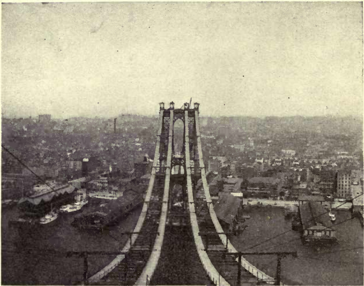
FIG. 47.—Manhattan Bridge. Footbridges and Sheave Towers.
