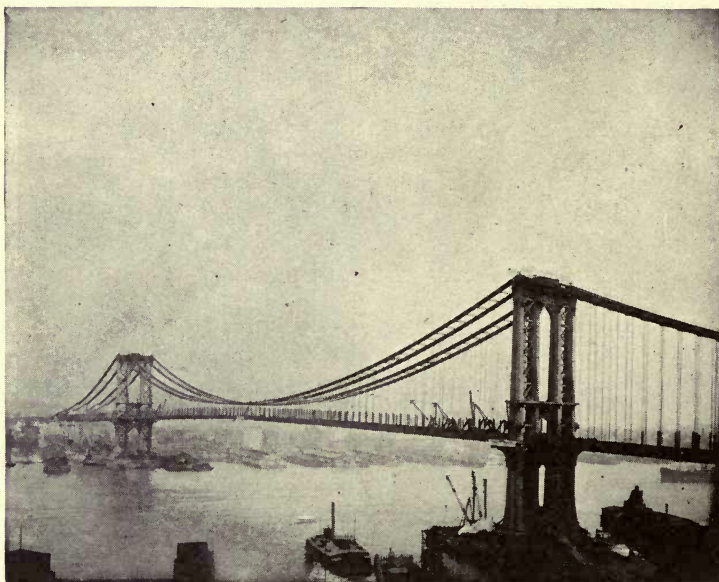
FIG. 52.—Manhattan Bridge. Erection of Diagonals.
