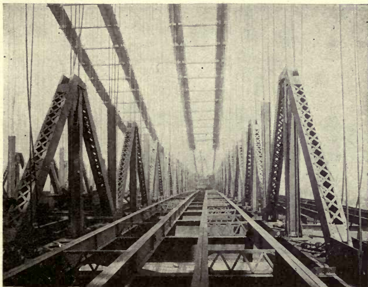
FIG. 53.—Manhattan Bridge. View before Erection of Top Chords.
