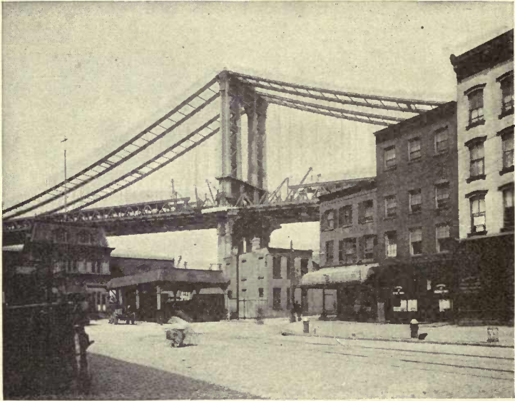
FIG. 54.—Manhattan Bridge. Erection of Top Chords.
