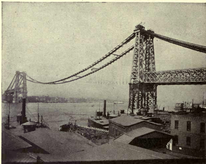
FIG. 57.—Footbridges for Erection of Williamsburg Bridge.
