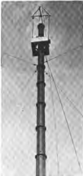
Fig. 314—Showing the Cage and the Top Mast Several Hundred Feet from Earth.
