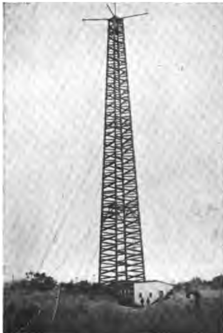
Fig. 300X—Wireless Station Erected at Cape Hatteras, N. C., U. S. A., in 1902.
