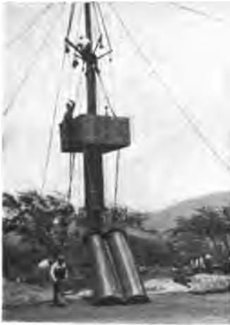
Fig. 312—Showing Workmen's Cage Which is Carried to the Top During the Process of Erection.
