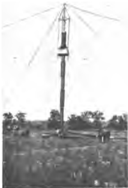
Fig. 313—A Tubular Mast in Early Stages of Construction.
