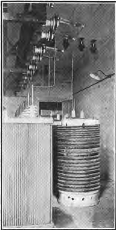
Fig. 307—Bank of High Voltage Trans-formers at Carnarvon Station. Fig. 308—The Switchboard of the New Brunswick High Power Transoceanic Station.
