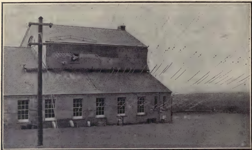
Fig. 303—Power House of the Trans-Atlantic Marconi Station at Carnarvon, Wales.
