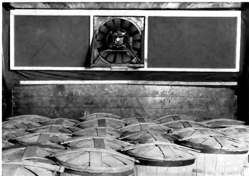
FIG. 1.—ELECTRIC FAN IN POSITION AT END OF CAR
