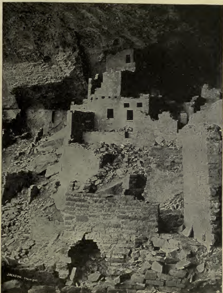
VIEW SHOWING TERRACES AND DIFFERENT STORIES.
