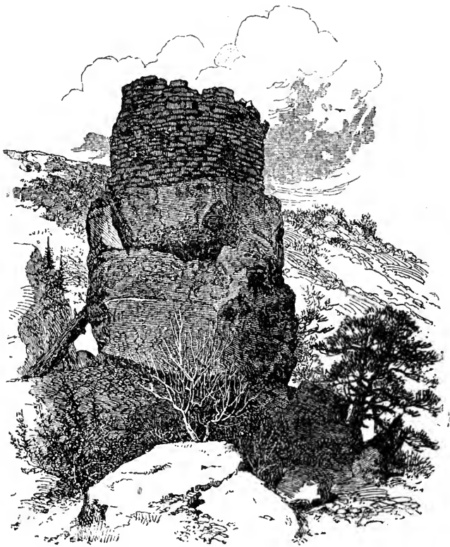
FIG. 2. BLACK TOWER ON THE MANCOS
