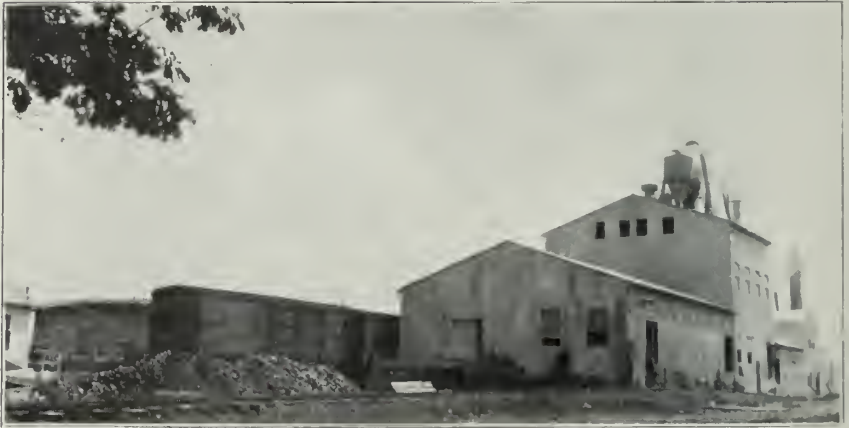
FIG. 3. The mill of the Standard Oil Company of Indiana, Olmstead, Illinois
