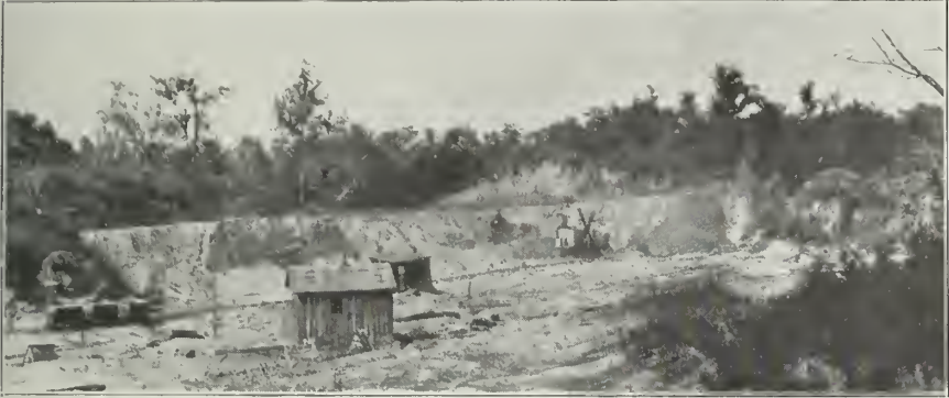
FIG. 6. The mine of the Sinclair Refining Company, showing the method of loading, the overburden, and general character of the deposit. Olmstead, Illinois.
