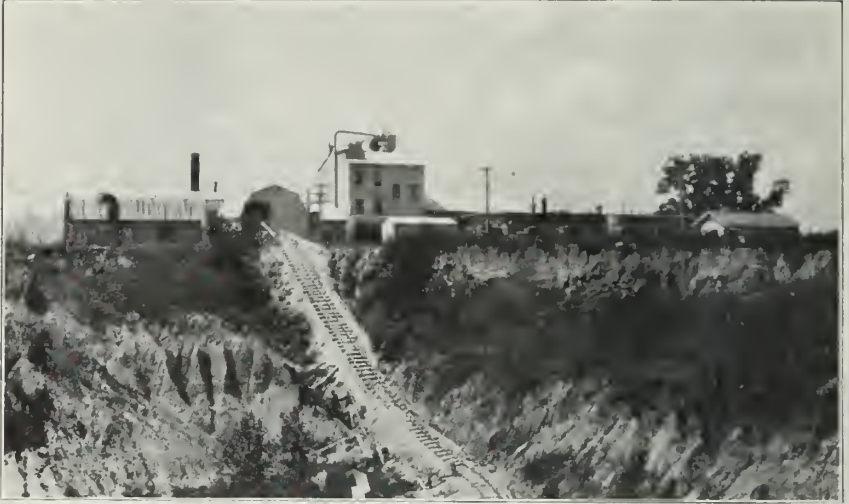
FIG. 2. The mill and incline to the mine of the Standard Oil Company of Indiana, Olmstead, Illinois
