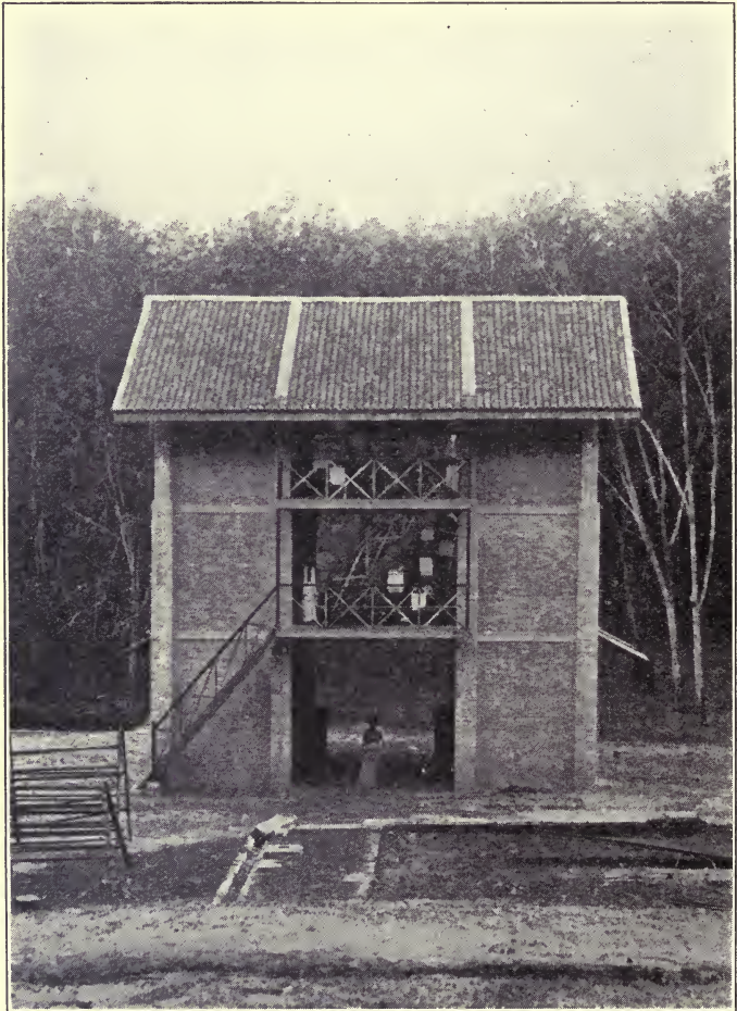
DOUBLE "DEVON" SMOKE-HOUSE OF BRICK, WITH ROOF OF CHINESE TILES, SHOWING LOADING PLATFORMS WITH RACKS WITHDRAWN FROM SMOKING CHAMBERS.
