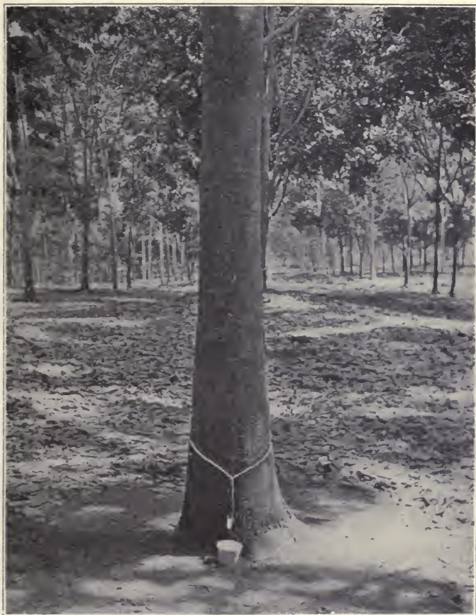
A V-CUT ON HALF THE CIRCUMFERENCE.
