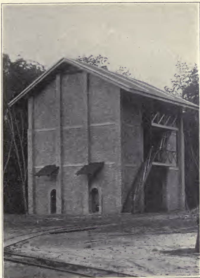
SIDE VIEW OF PRECEDING PHOTOGRAPH, SHOWING EXTERNAL ARRANGEMENT FOR STOKING FURNACES.
