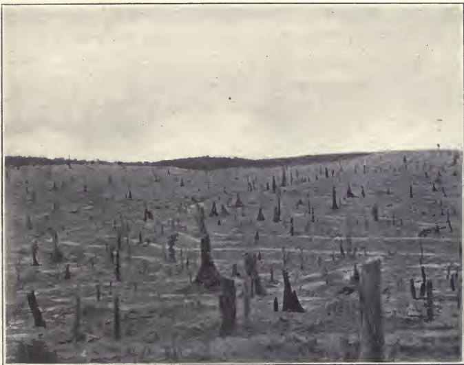
CLEARING READY FOR PLANTING.
