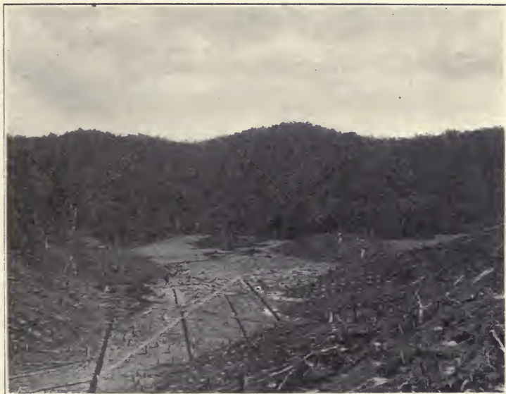
NEW CLEARING; SLOPES "HOLED" FOR PLANTING; FLAT AREA BEING DRAINED.
