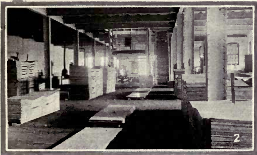
1, 2 and 3.— Creosoted wood block floors in the Follansbee Tin Plate Co., Follansbee, W. Va. These floors must withstand the wear and tear of heavy trucking
